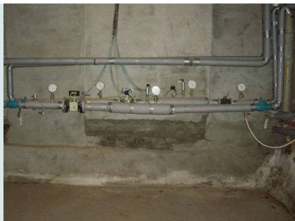
Photo-7: The basement of the multi-apartment house became dry and clean of unpleasant stench and breeding of mosquitoes, absence of water supply and heating in the apartments.
